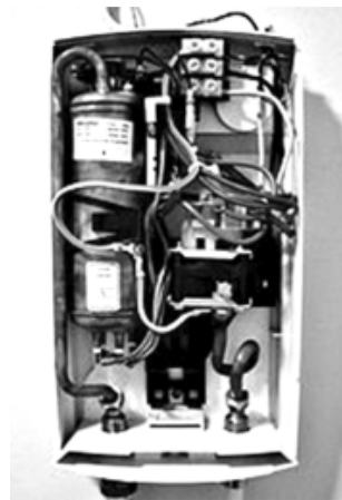
d) Tank-less Electric Water Heater
