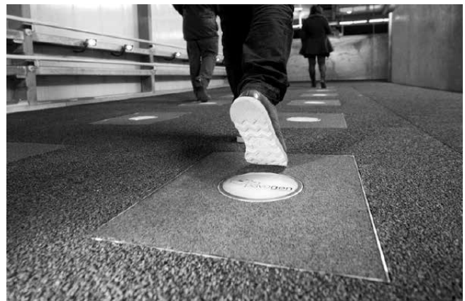
Figure 8: Experimental use of piezoelectric floor tiles. (C. Scholer et al. , 2009)
