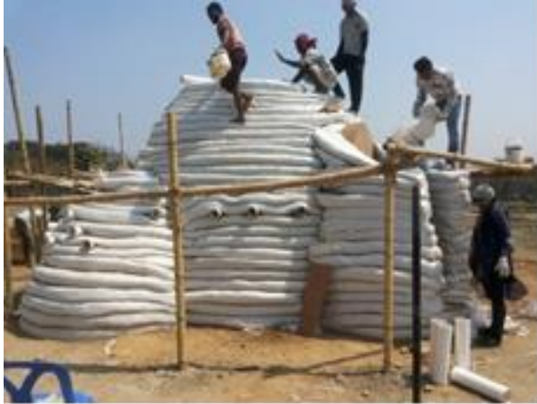
Figure 6: Step-7: (a) Repeat the process and completed dome
