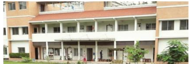
Figure 5: Building 1 (View from South)
