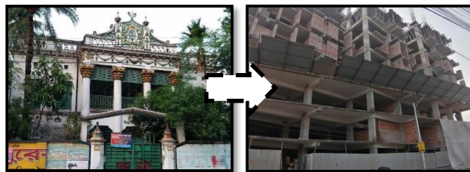
Figure 5: Before and After Jamidar Bari (Upper Jessore Road)
