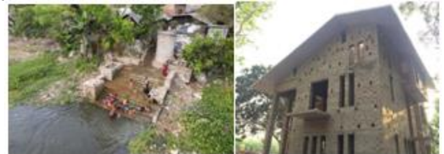
Figure 37:The project comprises two 'ghats' - stairways leading down to platforms in the river, with adjacent walkways - and the opening of previously obstructed footpaths that now lead to them.Simplecontextual designs.Housing Project in Jhenaidah, Photo: Bengal Institute, https://bengal.institute/news/kabir-an-architect-of-the-life-world/
