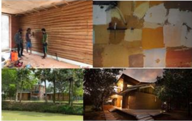
Figure 35: Mud wall, Shubarnadighi ,Client:Brigadier Baker, Gazipur, now being used as a resort. Rainwater filter system installed, gained Berger awards, tinned steel structures on the roof. He says, "The mud house needed a hat on head& a boot on feet to ensure safety from rain or storm water. As binding material he uses lime,shurki,thatch,Gum of trees, powder of leaves,cowdung, cheese etc from nature.
