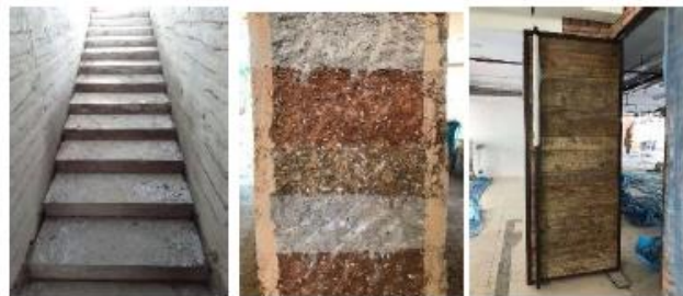
Figure 36:Mud made stair,discovery with different mud color ,use of raw wooden door. (courtesy: Mr. Nime)
