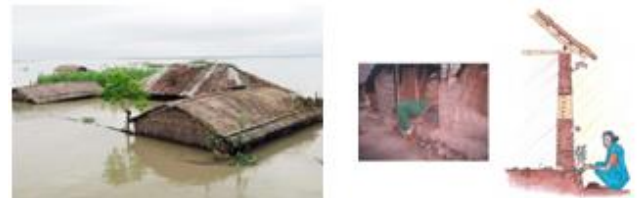
Figure 12: Flood situation worsen in BD,source-observerbd.com&traditional houses face various problems huge maintenance, damage by rain, flood& vermin infestation.[15][1][17] [5]
