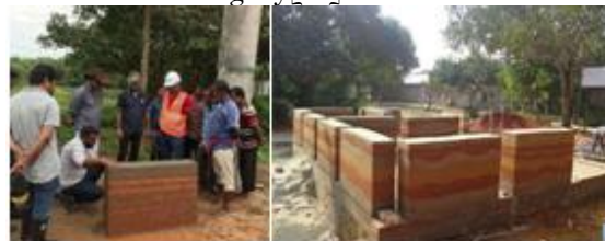
Fig52.Rammed earth formation source: Abdun Nime ,Earth constructor
