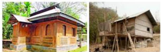
Figure 10. Bamboo & wooden house exm..Marma House - Bandarban, BD & Century old Momin Jame Masjid in Mathbaria, The entire structure of the century-old Momin Jame Masjid was made of wood in 1903 Pirojpur,source:TheBuisness Post19dec'21
