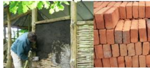
Figure 50: Abode brick picture &wattle construction process, Source:www.clovisstone.net&www.lowimpact.org[17]
