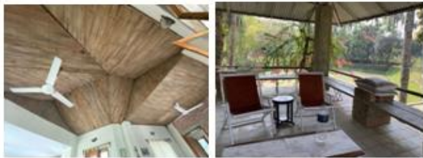
Figure 38- Beautiful vacation house with brick landing stage, Split Bamboo pith, frame remains hidden inside. Pavilion like in between space. Indoor outdoor relationship. Source –survey pic of Priyanka,(curtesy: Mr. Lutfur)
