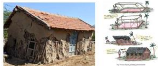
Figure 13: planetcustodian.com/mud-house-pros-and-cons & Cross-bracing of bamboo structural frame (adapted from Chishun 1979) To maximize benefits, adopt proper techniques, integrate local materials with modern technologies, and prioritize research for durable, sustainable vernacular architecture.[23][1][17][5]
